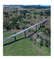
Butters Bridge is a true demonstration of innovative thinking. It boasts dual functions, conveying a 600mm diameter sewer, and provides a pedestrian and cycling link across the Molonglo River corridor. Rising to 27m above the river, the 242m long bridge is a vital piece of
