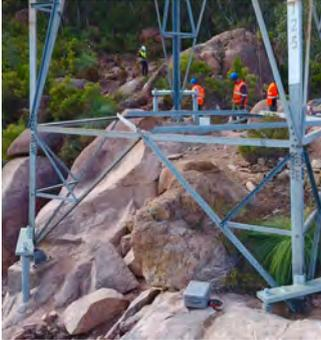
Transgrid transmission line number 970, forms a 132kV link between Burrinjuck and Yass substations in regional NSW. Concerns were raised by Transgrid engineers regarding the structural adequacy of the footings at lattice towers T125 and T126 adjacent to Burrinjuck
