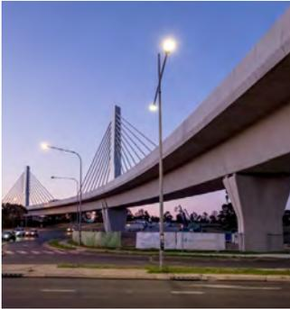
Located in the north west of Sydney is a unique, curved in plan, three-span cable-stayed rail bridge constructed using precast segmental concrete. The bridge is known as the Windsor Road Single Span Crossing (WRSSC) and it forms the tail end of a 4.5 km elevated viaduct that is part of the new
