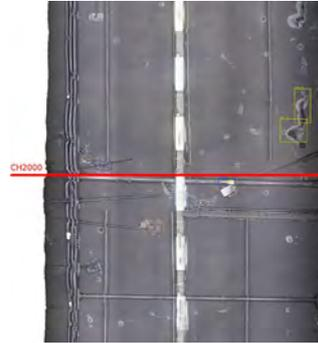
Current condition assessment practices of road tunnel ceilings involve manual inspection in difficult, time constrained conditions. Abyss Solutions has successfully demonstrated the capability of a new improved inspection method which combines high-resolution imaging
