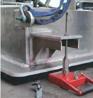
In the challenging environment of the Cook Strait New Zealand the OMV Raroa FPSO developed several through hull corrosion pits. Pushing the limits of conventional cofferdam repairs AMOG developed a highly economical solution which would achieve long term repair
