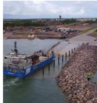
The Multi-User Barge Ramp Facility is a unique marine logistics facility at East Arm, Darwin, that is designed to cater for everything from Defence's beach landing craft to the 824 DWT Bhagwan Roller barge, and load any type of cargo including two 68 tonne Abram's Tanks concurrently. To meet
