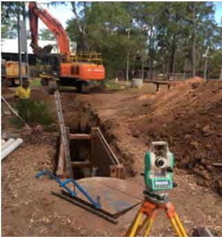
This is a project to replace the existing asbestos cement CED system with new gravity sewerage reticulation system. The site of work is at Angurugu Aboriginal community located about 630km from Darwin.
