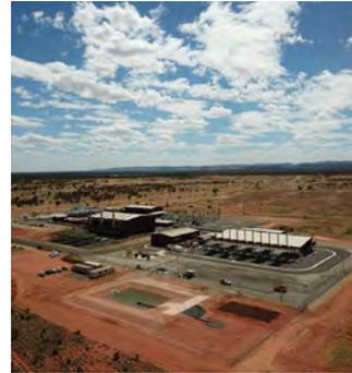
The Owen Springs Power Station (OSPS) expansion project is the construction of a nominal 44 MW gas fired power station including all required mechanical, electrical, controls and civil/ structural and balance of plant.
